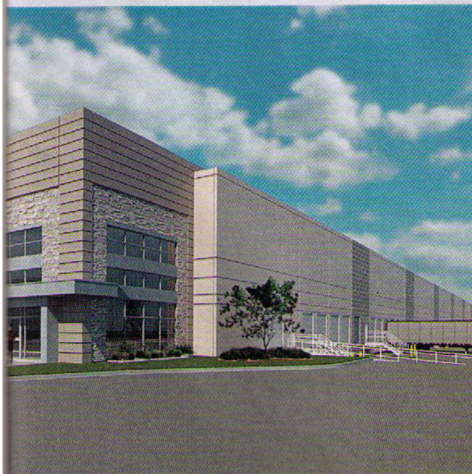
Construction on a 44-acre industrial park in Irving. The two buildings will total 537,300 square feet.
