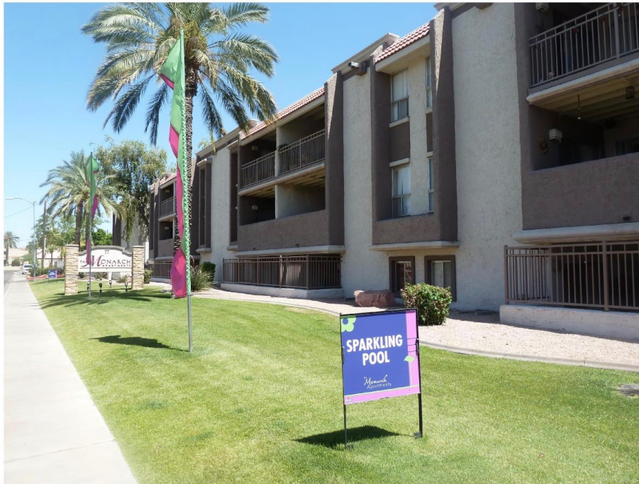
The Monarch apartments is located at 77 W. Coolidge Street in Phoenix. It is one of the 12 multifamily assets included in this refinancing.
