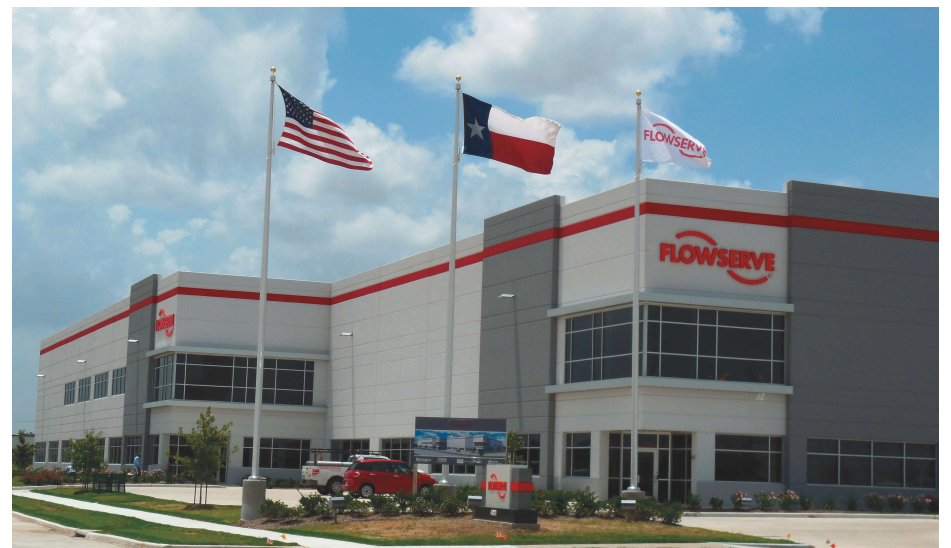
In Pasadena, this 95,000-square-foot FlowServe Corp. facility will serve the company's valves and seals division, and an adjacent project will house the pumps division.
